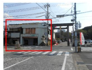
①Pocket park before construction
